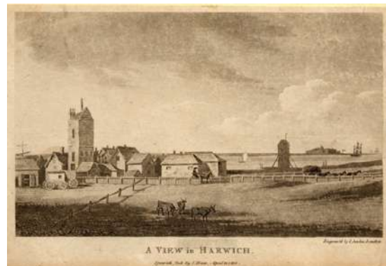
Figure 7 A view in Harwich, 1808, prior to the building of the low and high lighthouses in 1818 (ERO X172-19 Imp 170-1-27)
