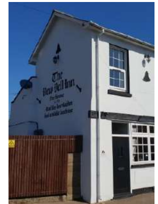
Figure 31 The New Bell Inn
