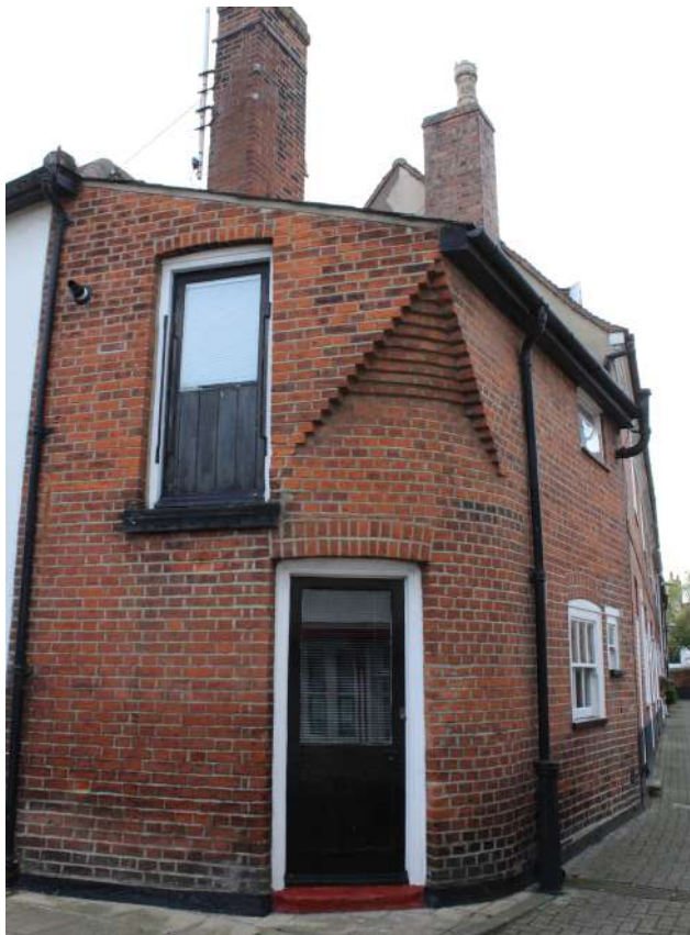
Figure 37 Building detail on George Street
