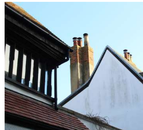
Figure 18 Example of varied roof scape
