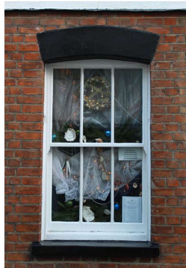
Figure 24 Decorated Window in Harwich
