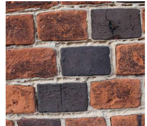
Figure 17 Red brick within the Conservation Area
