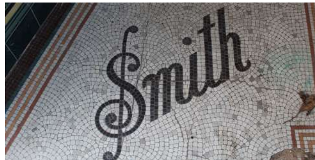
Figure 41 Tiling on Market Street
