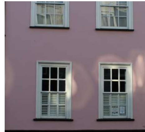
Figure 16 Example of Georgian facade
